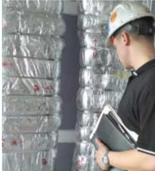
fire protection of grease ducts, four small shaft walls are constructed to enclose the duct. This configuration is assumed to provide equivalent protection to that of the flat, full size shaft wall. While code compliant, a fire rated shaft wall is *not a tested system* for grease duct enclosures.
